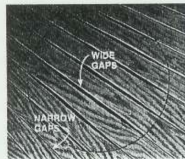
FIGURE F WHAT CAUSED THE GAPS in this solid wood floor? And why are they only in this small circular area? (Give up? Check the end of this article.)
